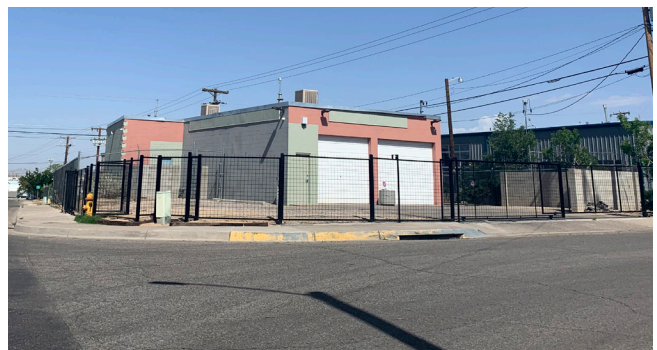
Typical industrial development at Prospect Avenue and Quincy Street.
